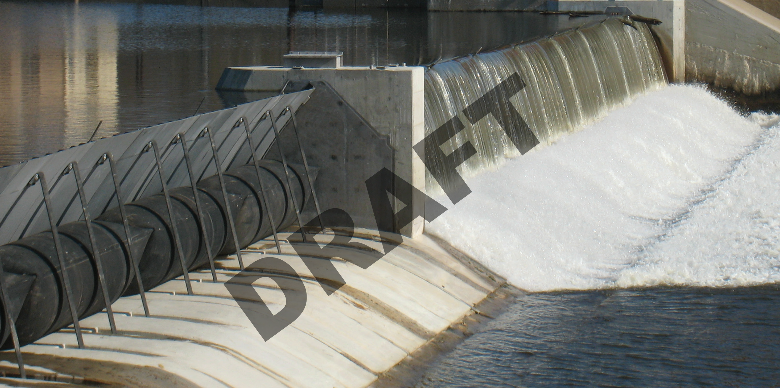
Inflatable Adjustable Weir
