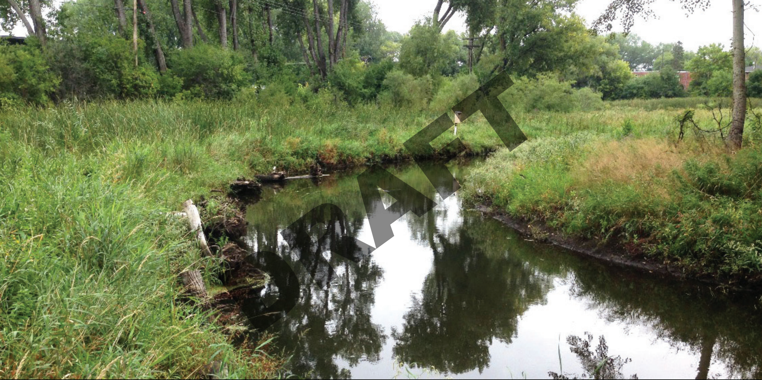
Bioengineered Bank at Minnehaha Creek, St. Louis Park, MN
