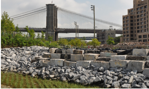
Stone Blocks (1-1.5m W x 1-4m L x 0.75 m H)
