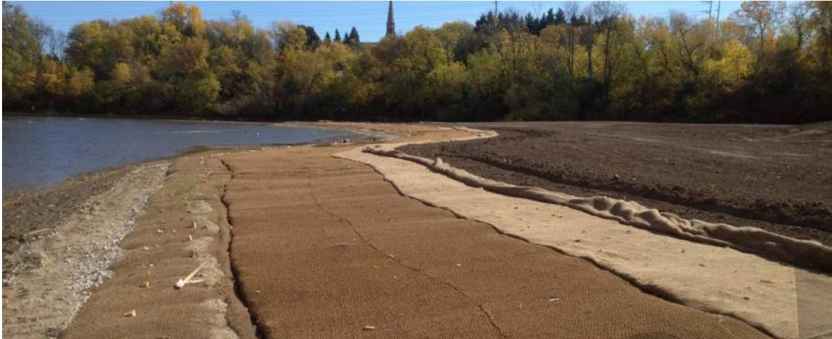
**Fabric Encapsulated Soil and Gravel Lifts**
