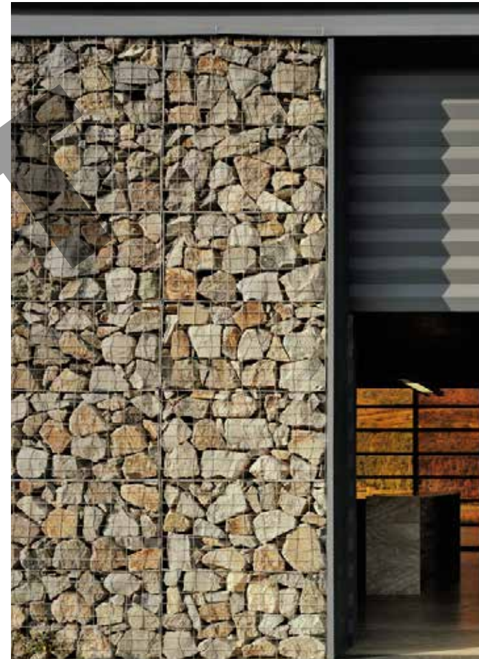
gabion wall aluminum-framed glazing
