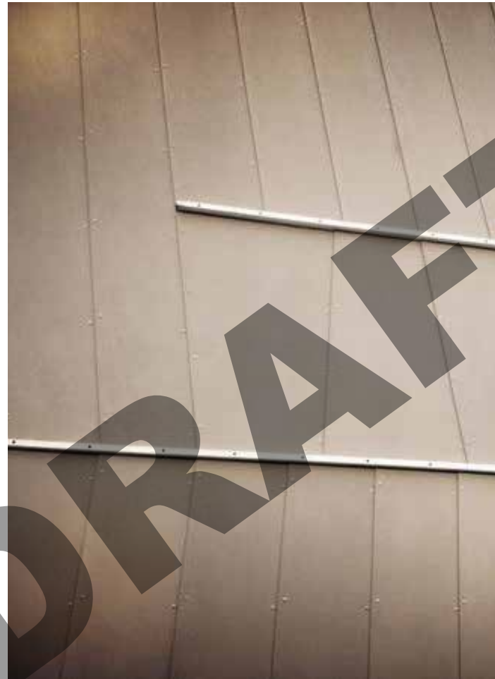
solid phenolic panel soffit
