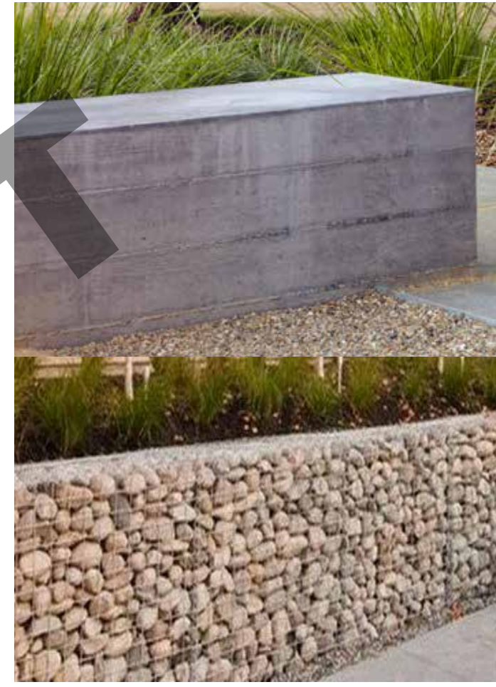
concrete retaining walls/gabion
