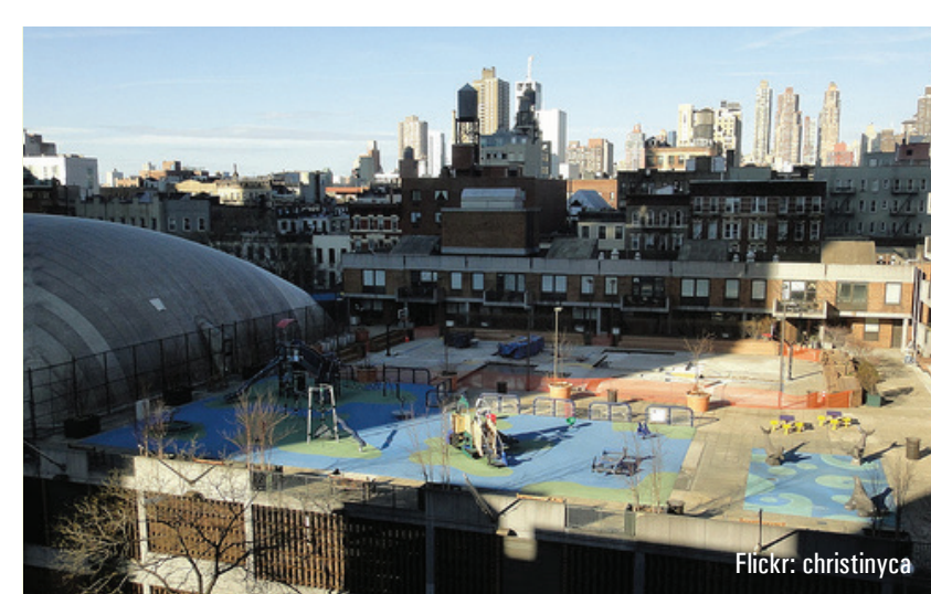
Manhattan Plaza Apartments, New York An affordable housing complex that includes a rooftop playground and a pre-school facility.
