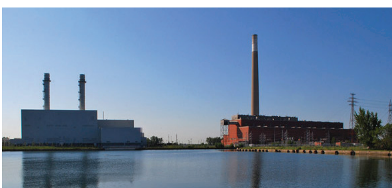
The Hearn and Portland Energy Centre
