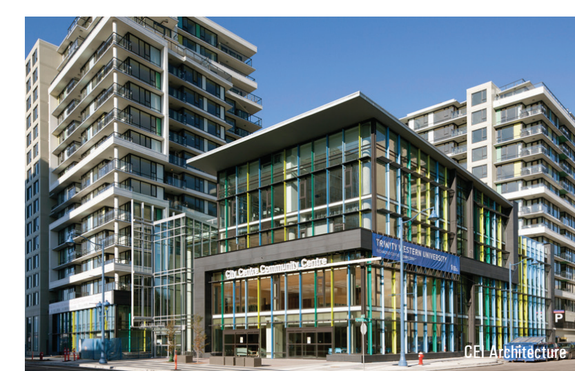
City Centre Community Centre, Richmond, BC Community centre in a five tower residential and commercial mixed use development.
