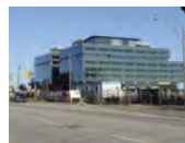
CORUS QUAY Type: Commercial/Industrial Length: 90m Depth: 85m Floors: 4 Floor Plate : 7650m2
