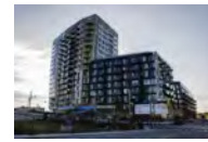
WEST DON LANDS Type: Residential/Mixed use Length: 100m Depth: 72m Floors: 8-15 Floor Plate : xm2
