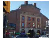
ST LAWRENCE MARKET Type: Commercial Length: 105m Depth: 46m Floors: 4 Floor Plate : 4830m2
