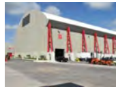
PINWOOD MEGA-STAGE Type: Commercial/Industrial Length: 60m Depth: 80m Floors: 4 Floor Plate : 4800m2
