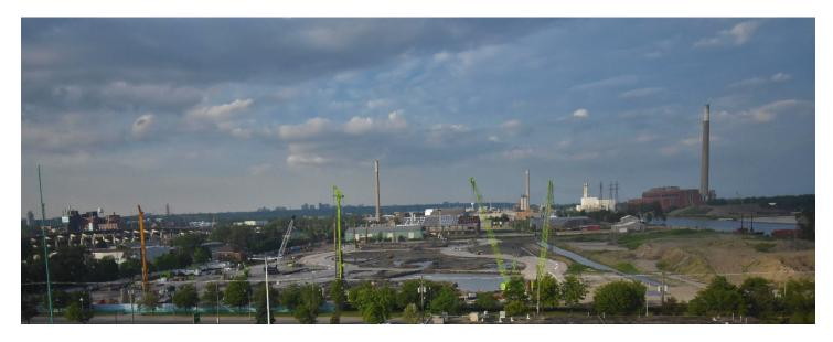
Excavation continues on the first section of the new river valley. We are installing watertight retaining structures (called secant piles) along the edges of the new river valley. These piles support the cut-off walls that will keep the excavated area stable and dry as work progresses. Looking east across Cherry Street, temporary access roads make it easy to see where the future location of the northern and southern banks of the river valley.
