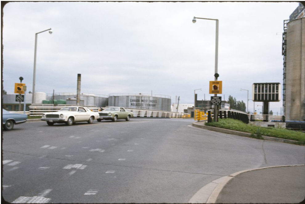
1968 bascule bridge, photos taken in 1976 (City of Toronto Archives).
