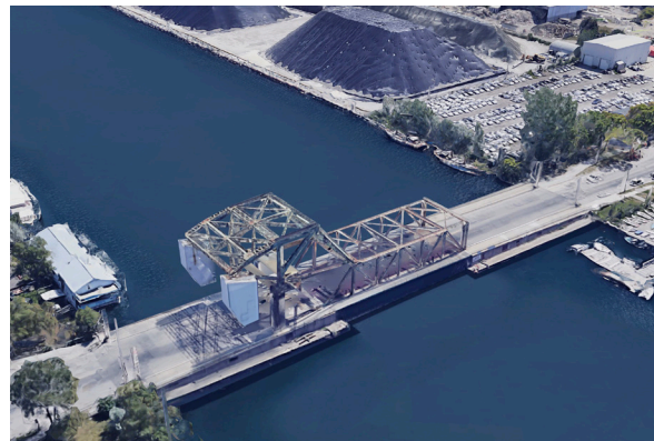
South Cherry Street Bridge (Google Earth, 2018).
