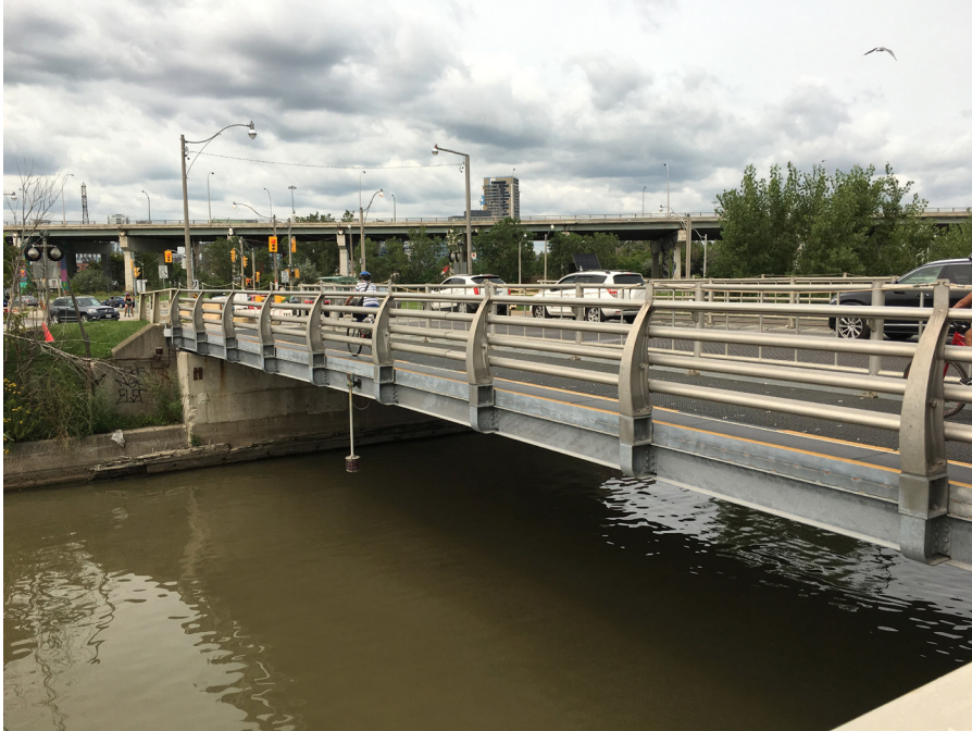
Looking northeast toward the Bridge (ERA, 2018).
