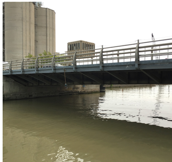
Steel deck as viewed from the northeast (ERA, 2018).
