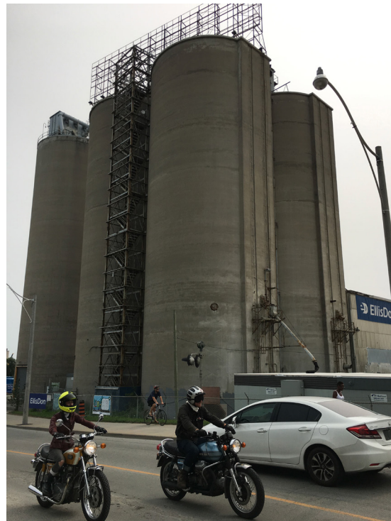
Century Coal Company silos at 312 Cherry Street (ERA, 2018).
