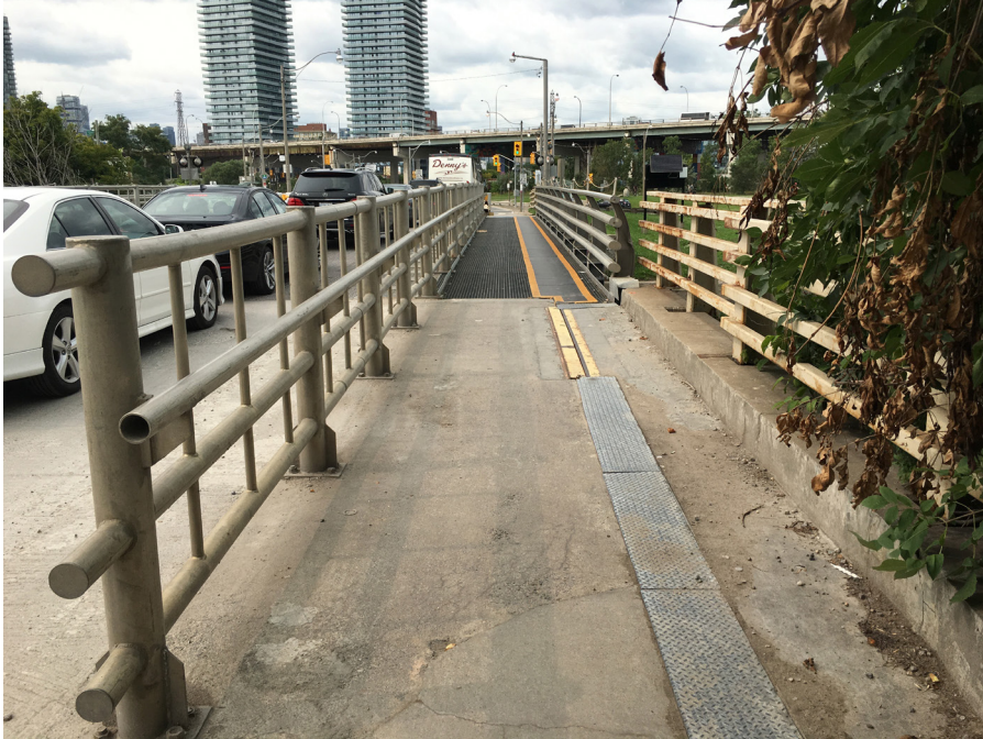
Looking north toward the Bridge (ERA, 2018).
