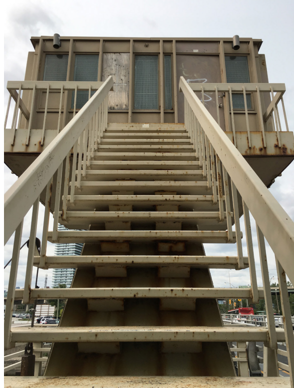
Operator's house and access stair (ERA, 2018).
