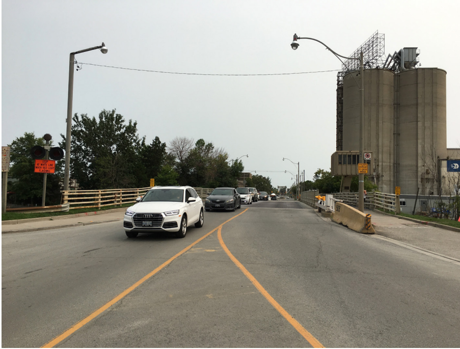
Looking south toward the Bridge (ERA, 2018).
