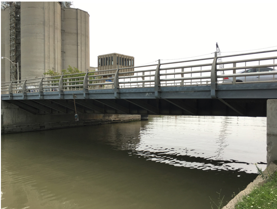
Looking southwest toward the Bridge and operator's house (ERA, 2018).
