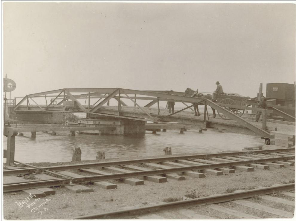
A steel swing bridge over Keating's Channel, c. 1898 (City of Toronto Archives).
