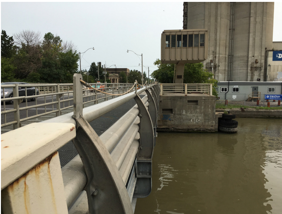
Looking south toward the Bridge and operator's house (ERA, 2018).
