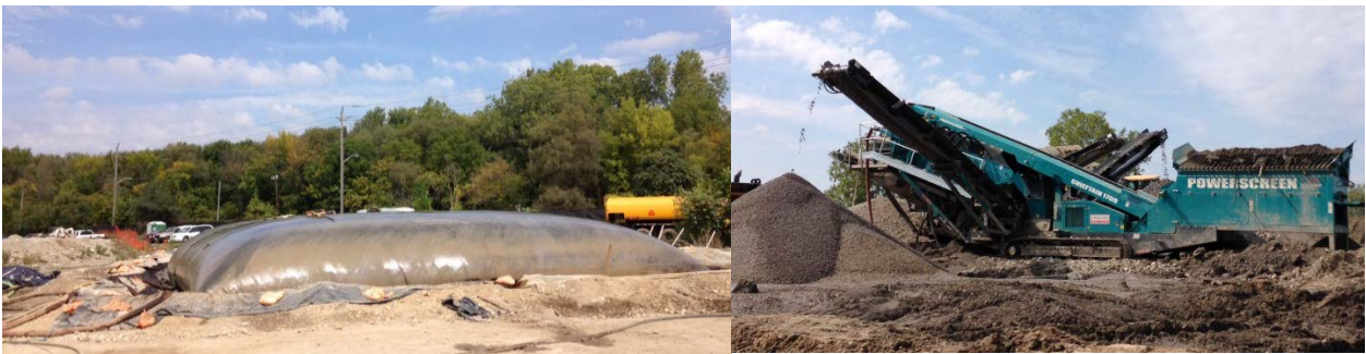
Photo 4. Example of Soil Washing, Soil Screening and Water Management
