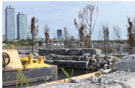
**Top:** A total 240,000 metric tonnes of clean, locally sourced material has been placed, shaped and packed around Essroc Quay.
