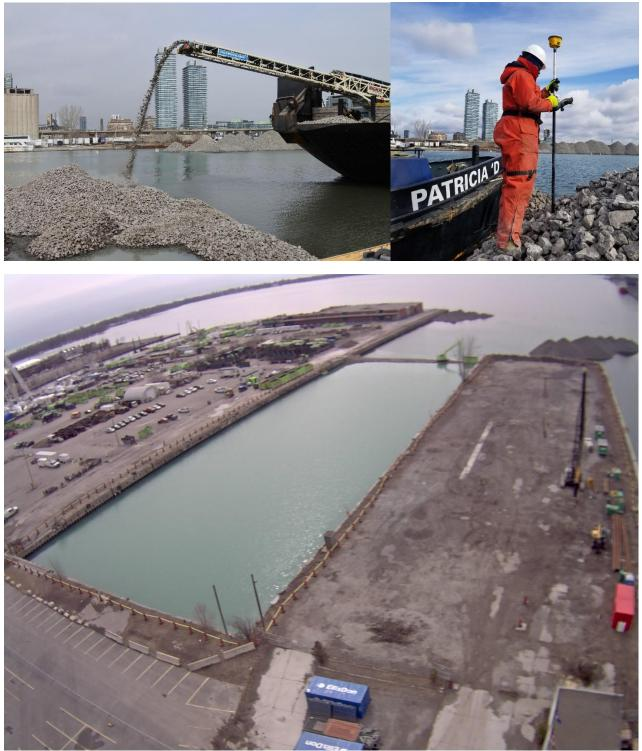
From left: Stone being placed in the Inner Harbour to form a berm, surveying of placed stone, view of the completed berm.
