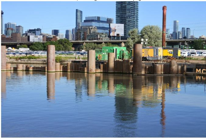
Crews have completed installing the pipe and sheet piles that will support the new dock wall. Later this month the crew will start to install the rock anchor, which will involve cutting the pipe and sheet piles, installing the casing and drilling. The drilling will be vibratory, which keeps noise to a minimum.
