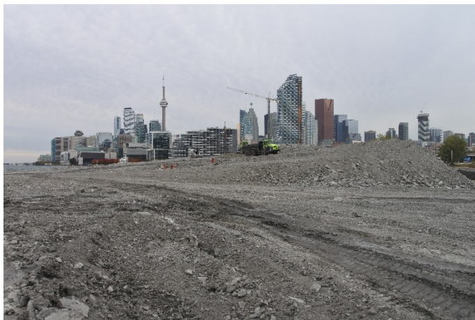
Lakefilling continues (left). A total of 19,560 truckloads of locally sourced clean fill, that will form the northwest corner of Villiers Island. The dock wall construction continues (right). The crew is placing rebar and forming the cap beam.
