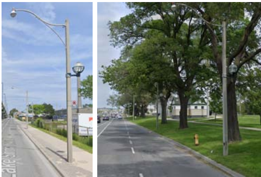
Existing Combined Roadway & Pedestrian Lighting on LSB Shared pedestrian and street lighting pole no longer permitted
