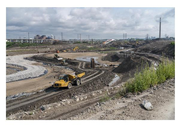
**Above**: In addition to river finishes, we're also installing pedestrian and cycling bridges in the river valley to connect trails through the wetlands that will line the main river channel. The tall vertical structure in the centre of this photo is part of the foundation for one of the pedestrian bridges.
