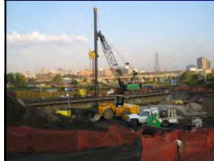
Initiate Shoring for Bala Underpass
