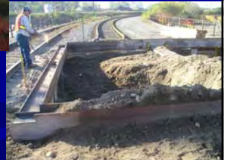
Begin Excavation of Elevated Rail Bed in Preparation for the Bala Underpass
