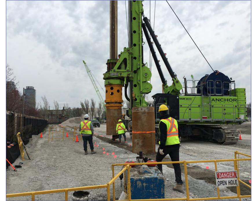
Drill rigs install a secant pile for cut-off walls that will help keep excavation dry and stable.
