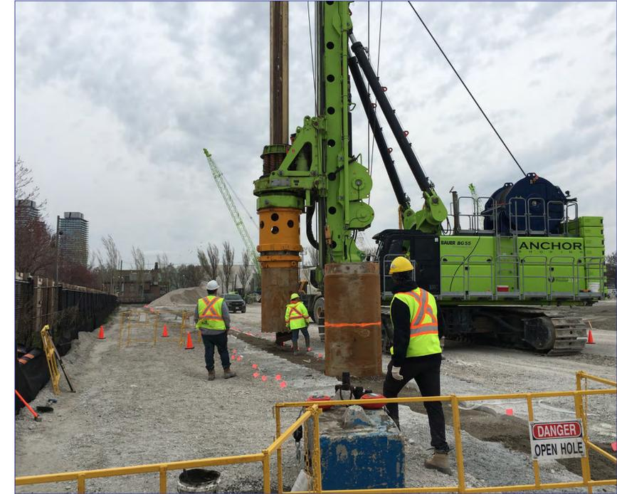
Drill rigs install a secant pile for cut-off walls that will help keep excavation dry and stable.
