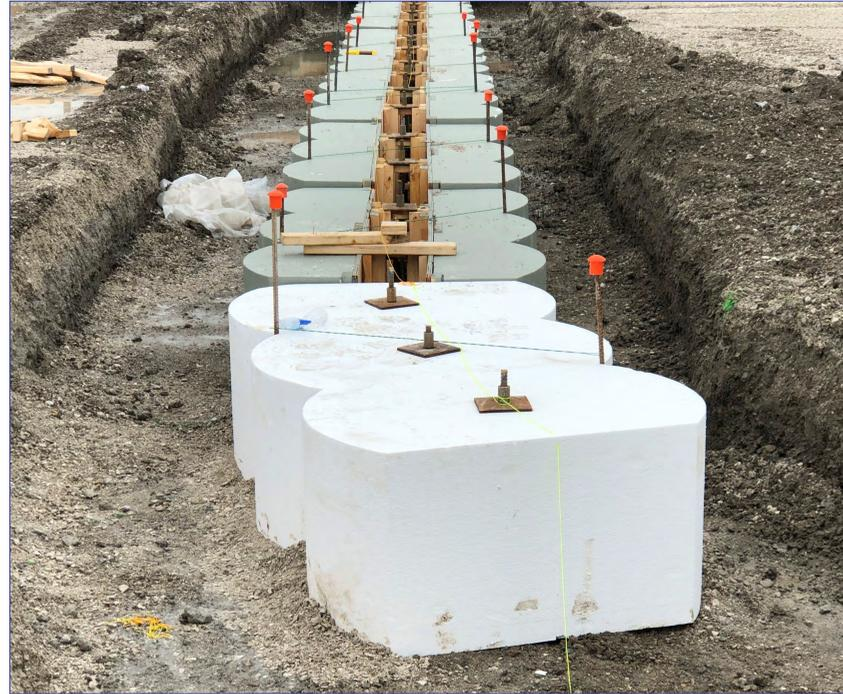
Guide walls line the edges of the new river valley as we prepare to install secant piles for cut-off walls.
