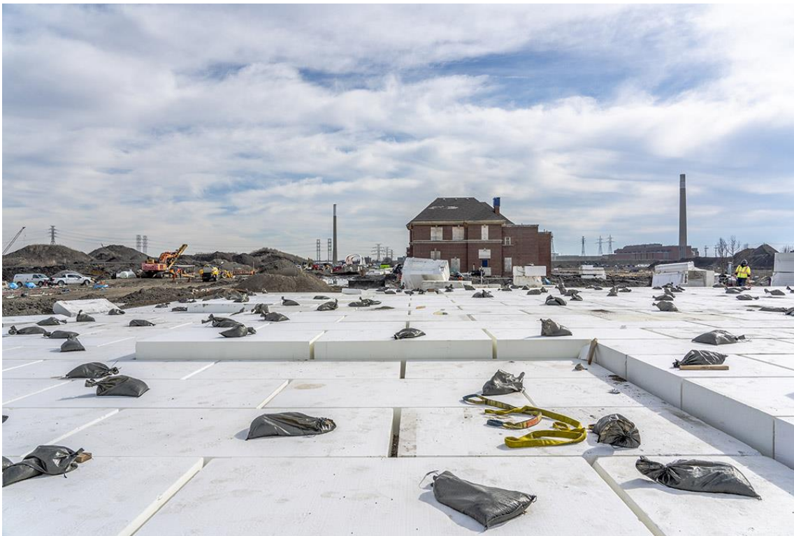
Above: These large white blocks are geofoam in future River Park North. This lightweight material is placed in the ground above infrastructure like pipes to avoid putting too much weight on them. Then the geofoam is covered with soil.
