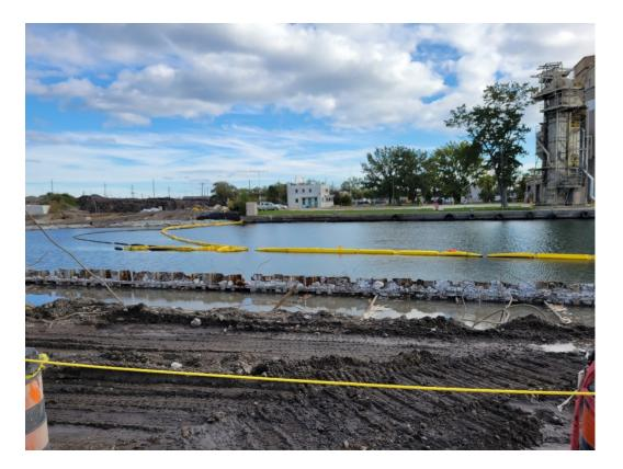
**Above:** This is the dockwall on the north side of Polson Slip – the future 'canoe cove', which will be where the new mouth of the Don River meets the lake. After adding underwater reinforcements to the dockwall last year, we're now excavating the area closer to the surface of the water to make the river mouth wider and also the create a place to launch small boats and islands to paddle around.
