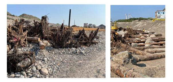
**Above:** These trees and rootwads were installed to protect the future riverbank from erosion and provide habitat for fish.
