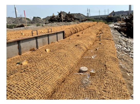
**Above:** These step-like layers are called 'fibre encapsulated soil lifts', and are used to make up the future river bank. Each layer has soil mixed with seeds wrapped with a special fabric to hold the soil in place while the plants get established. Eventually, the fibre wrapping will biodegrade and the plant
