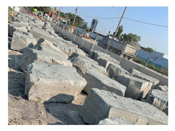
**Above:** These large rocks are 'armour stones' and destined for the new mouth of the Don River. Some of these stones will be placed underwater, so we line them all up and figure out which ones fit together best first.
