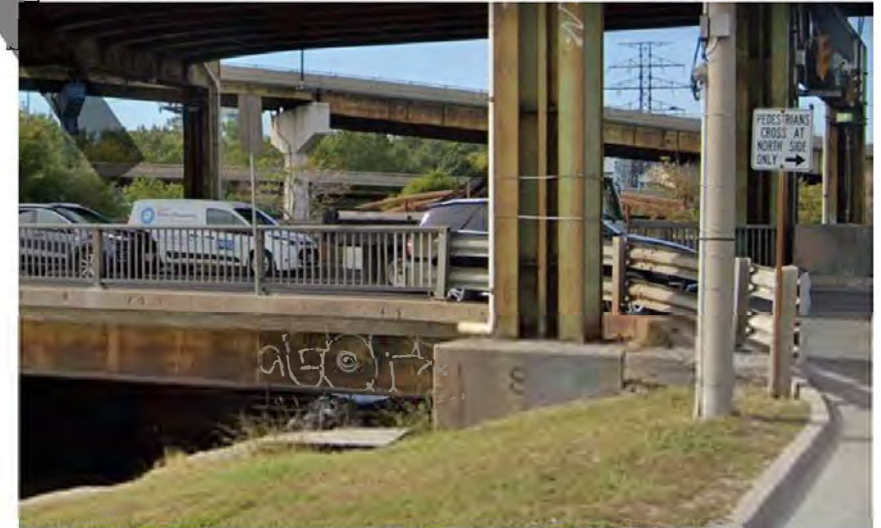
Existing Condition - Bridge and Bent at Intersection
