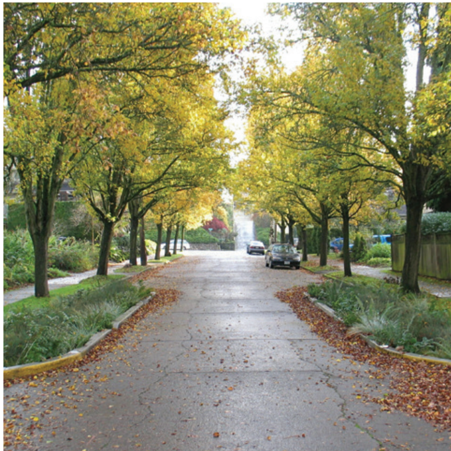
A residential green street with curb extensions and bioswales and mature tree canopy
