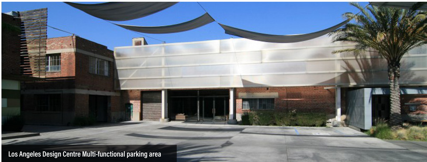
Examples of Surface Parking Lots and Structured Parking
