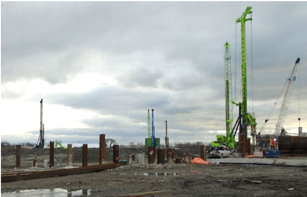
Above: Cut-off wall construction along the perimeter of the future river valley south of Commissioners Street just west of Don Roadway.
