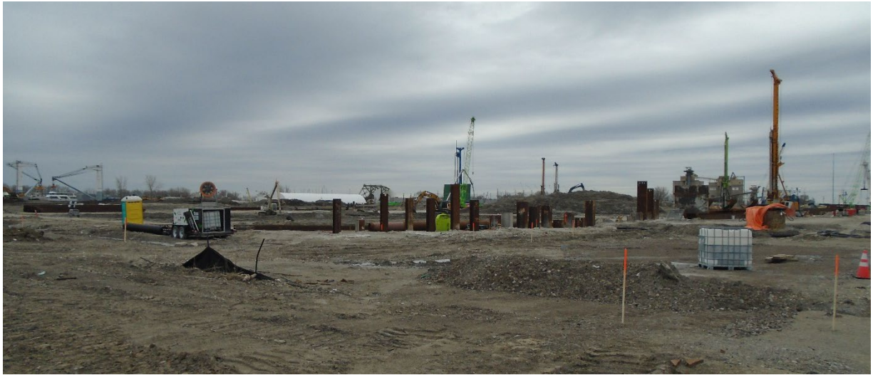
Above: Cut-off walls are almost complete in the first section of river valley, south of Commissioners Street just east of Cherry Street. Crews are now preparing to start deep excavation in this section.
