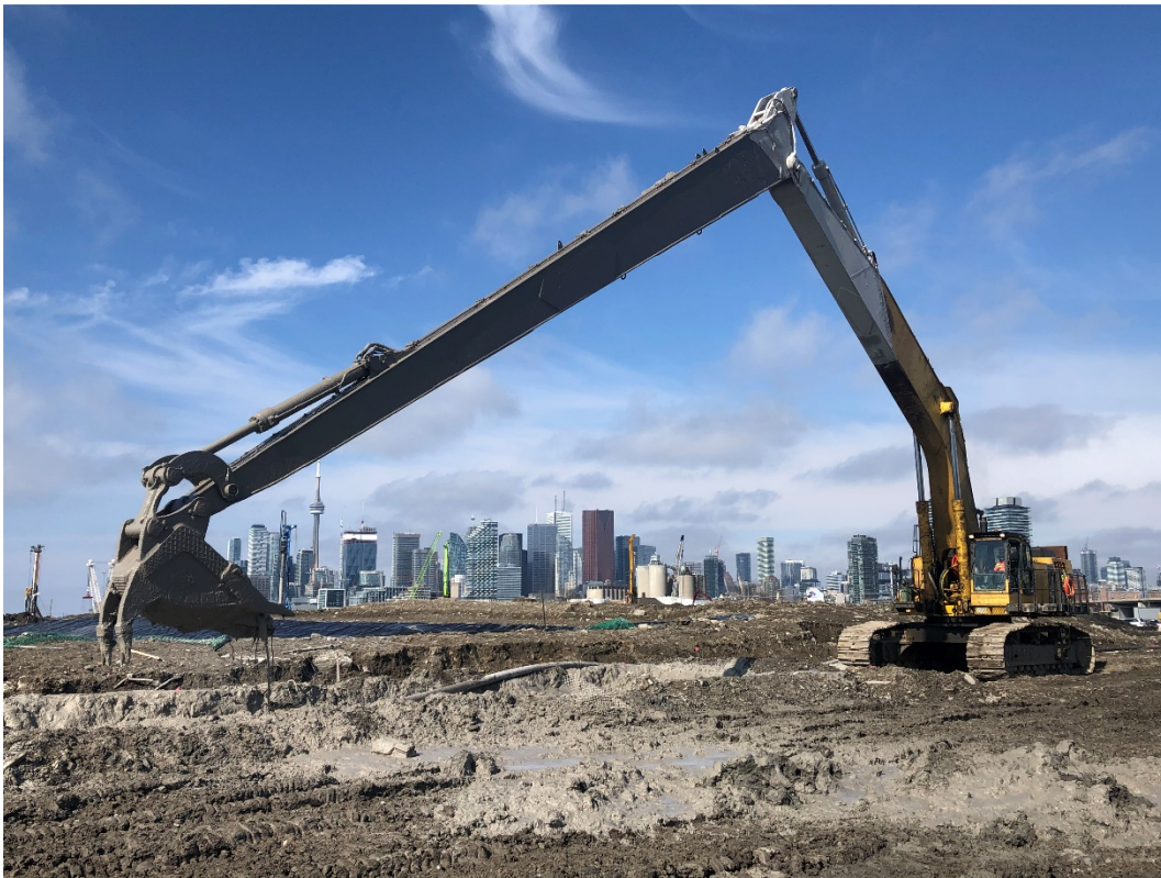
Above: Crews have started excavation in the second section of the river valley, just west of Don Roadway to the north and south of Commissioners Street. Rocky the Rock Ripper is making progress digging trenches for the slurry walls that will keep the area dry as crews dig the new river valley.
