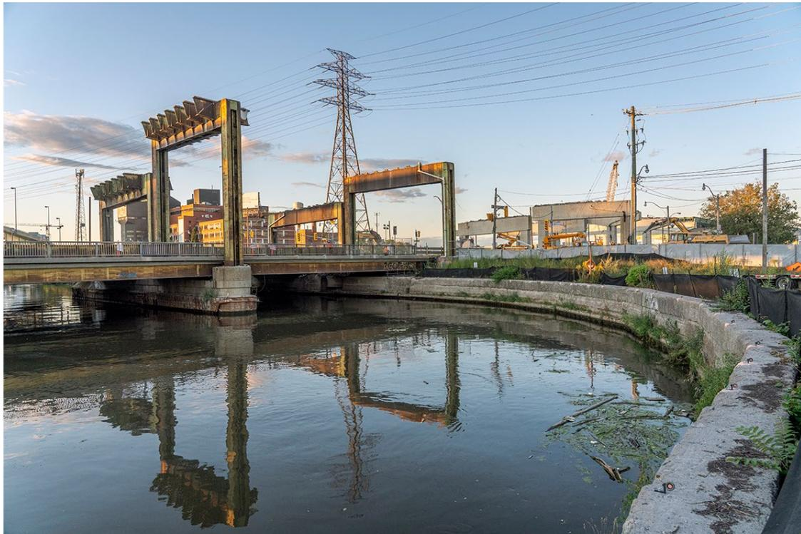
*Above: Looking north at the bend in the Don River where it meets the Keating Channel, you can see the road has been removed from the Logan ramps across the Don River. Once the overhead structure is gone, crews can safely widen the mouth of the Don in order to achieve flood protection.*
