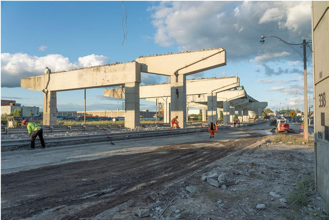
*Above: Crews made significant progress in the first weekend of work to remove the Logan Ramps from the Gardiner to Lake Shore. Looking west from Lake Shore, you can see where the deck has been removed.*
