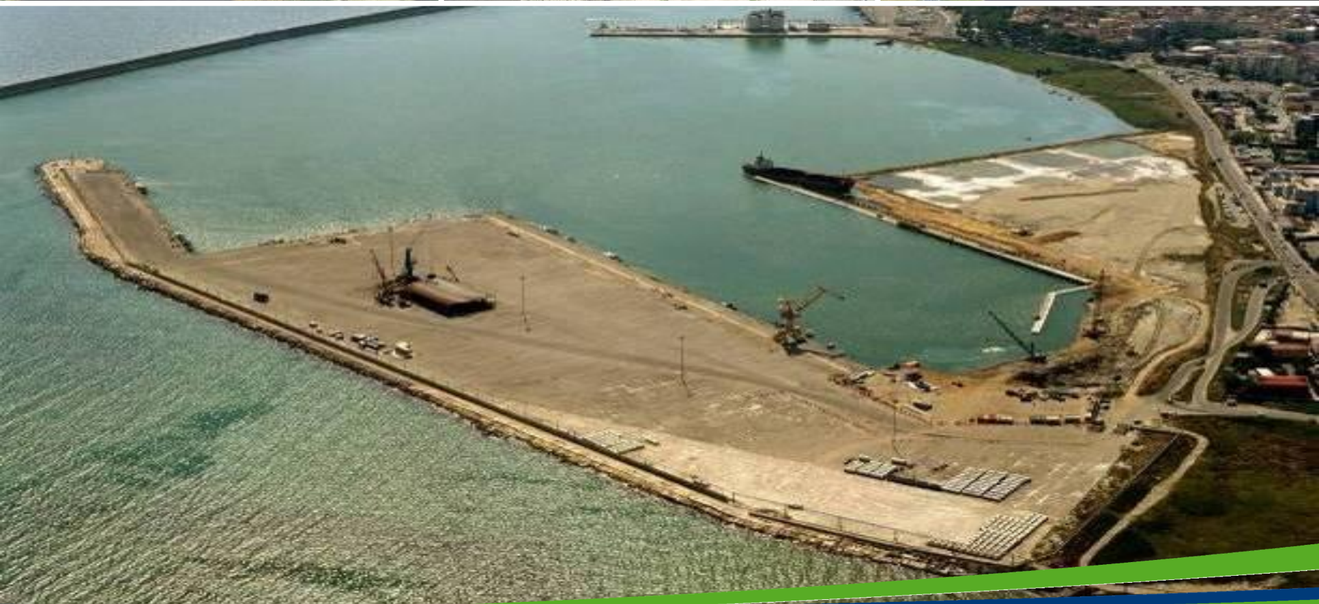
Sediment Treatment & Land Reclamation
