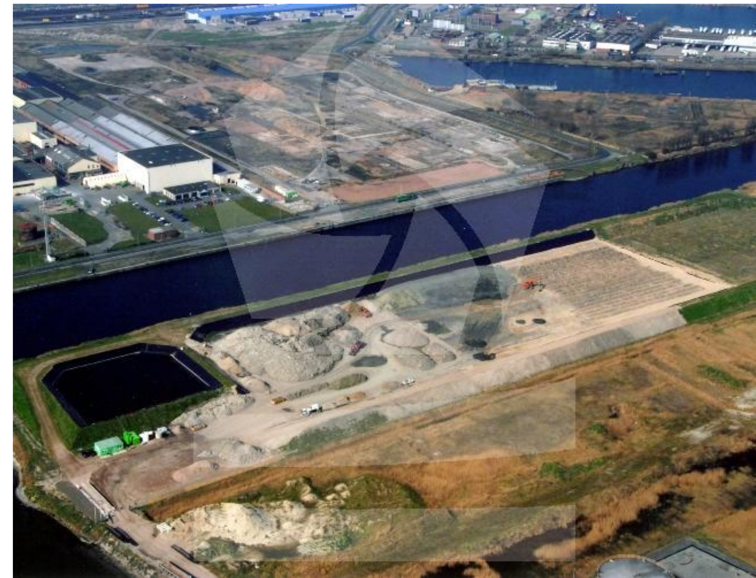
Soil Recycling Facility, Zeebrugge, Belgium
