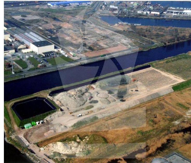
Soil Recycling Facility, Zeebrugge, Belgium
